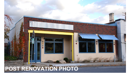
POST RENOVATION PHOTO
